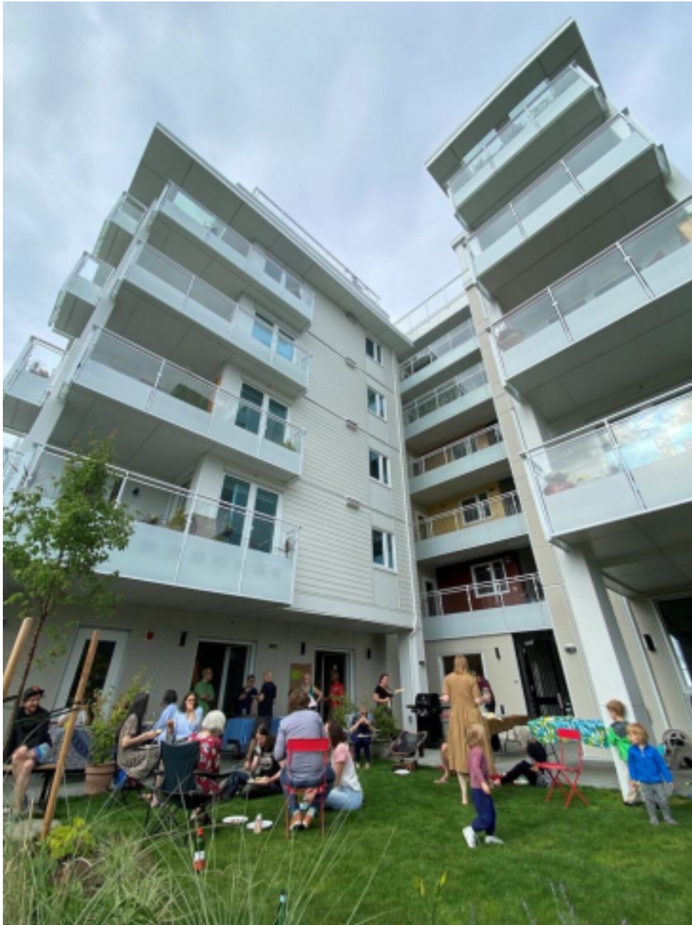
Little Mountain Cohousing community lives in a six-storey, multigeneration building in Vancouver.
